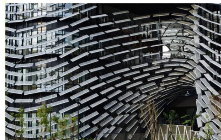
Industrial Technology Research Institute, Taiwan To form a wave second skin, to hide the facilities and to allow for expansion as research progresses
